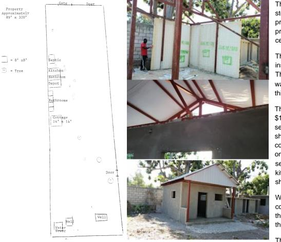
The walls are Styrofoam and steel and make it hurricane proof, earthquake proof, bug proof, and much cooler than cement blocks.
