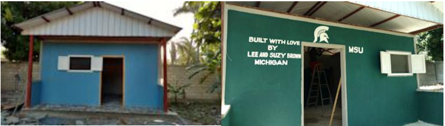
The blue house will say "BUILT WITH LOVE BY GRACE FOR HAITI -- NEBRASKA" when our artist-painter returns.
