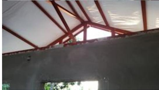
The hot tin roof has this special insulation to keep it cool.
