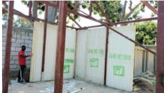
The walls are Styrofoam and steel and make it hurricane proof, earthquake proof, bug proof, and much cooler than cement blocks.
